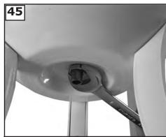
Install light fixture over all thread and use nut provided to secure in place.
